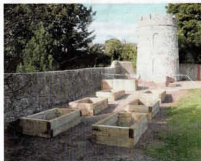
The finished compost bins and raised beds
